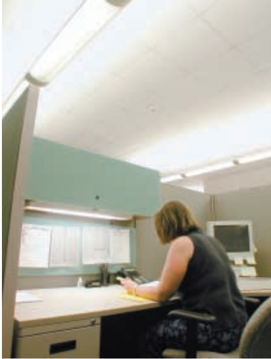
Task lights located underneath overhead storage bins triple the number of footcandles per desktop.
