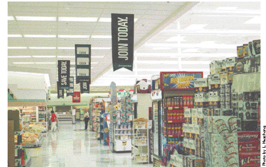
A raised ceiling pulls customers into the skylit center of this grocery. A conventional dropped ceiling rings the perimeter.
