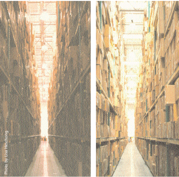
(Left) Metal halide fixtures produce dark shadows on boxes. (Right) Diffuse skylights provide better illumination on the box faces top to bottom.
