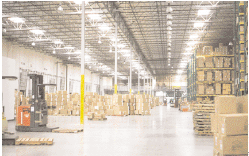
All the metal halide fixtures are turned off in the shipping and receiving area of a major warehouse. Note how the white walls and light colored concrete floor help distribute the daylight.
